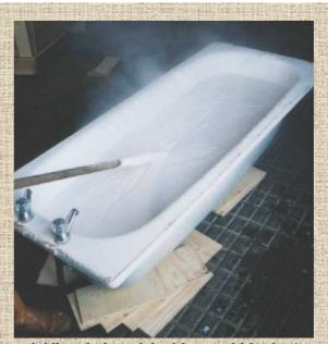
quicklime being slaked in an old bath: the lime must be added to the water and not the other way round, as it could cause an explosion. The ratio of water:lime is 3:1. To ensure that all the lime is slaked, the mixture is raked continuously for 10 minutes. There is a violent reaction, and heat and steam is given off. When it is cool, the 'lime putty' can be stored in plastic buckets indefinitely as long as there is a layer of water on top.
