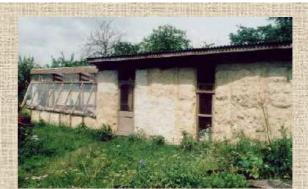
straw-bale building with lime render: 1 part lime putty is mixed with 3 parts sharp sand. The walls are sprayed with water first; apply two coats, and allow each to dry slowly by covering with wet sacking.
