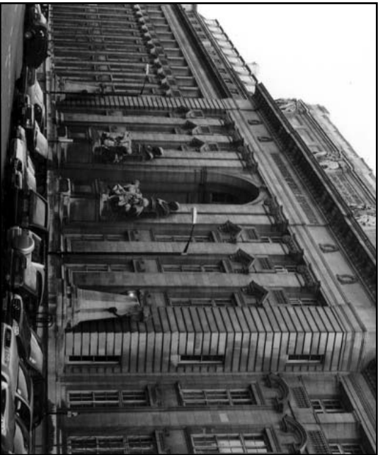
Imperial College London's Royal School of Mines, home of Centre for Petroleum Studies. Photo: Louise Sales
